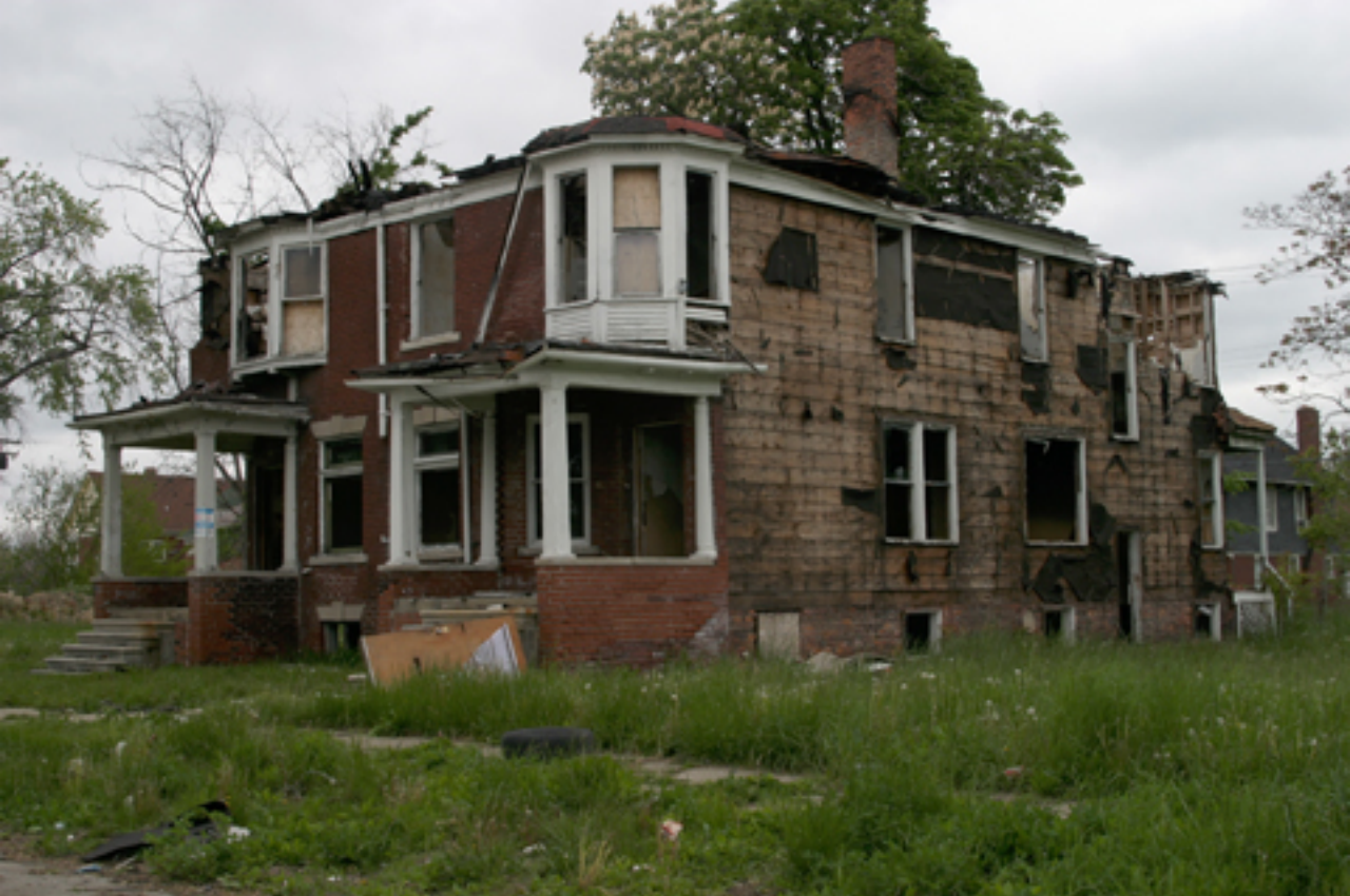
Abandoned house on Detroit's east side
